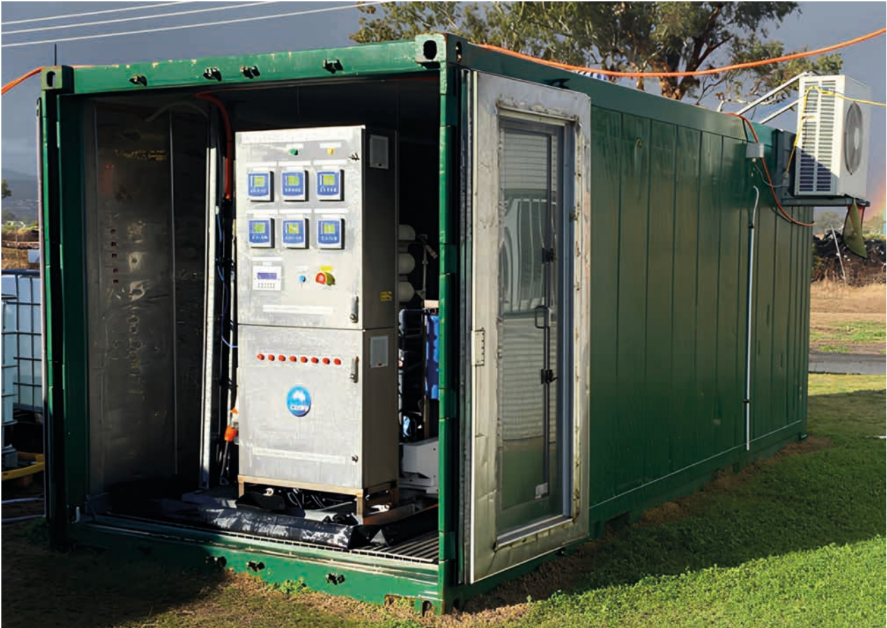
Figure 6. Water Corporations iFORO prototype fits in a 20-foot shipping container and can treat up to 10,000 litres of per day. Courtesy CSIRO.
