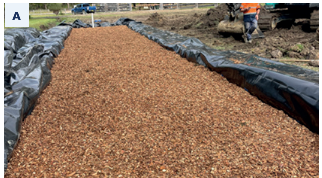
Figure 3. Construction of the bioreactor involved digging a pit 25m long x 4m wide x 0.6m deep (A) and lining it with thick black plastic (B) to prevent seepage of the runoff
