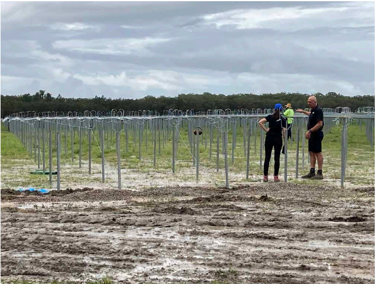
Richard McGruddy (R) showing Wendy Morris (L) the new tabletops in the final stages of installation at Queensland Berries. Photo credit: Mark Salter
