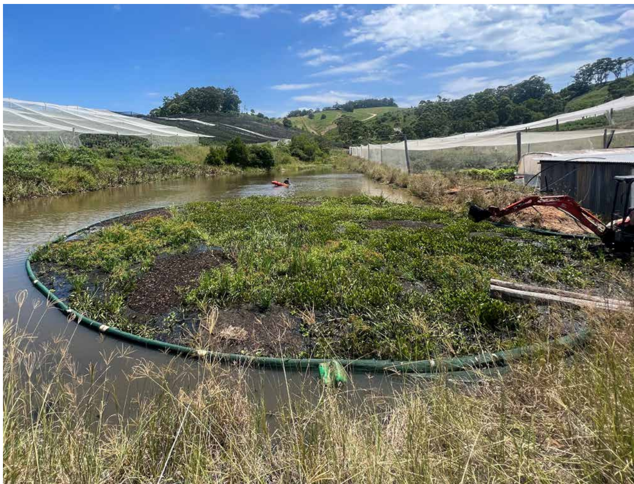
Figure 7. A net is used to clean up the remaining floating weed after the excavation has finished
