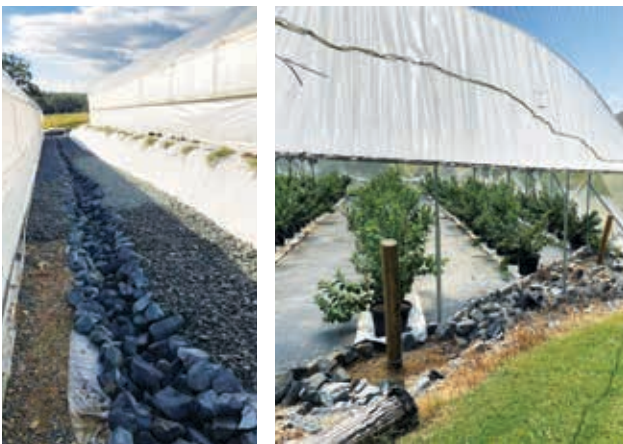
Figure 4. Erosion and run-off control through water being slowed as it passes through strategic placed rocks. Photo credit: Melinda Simpson
