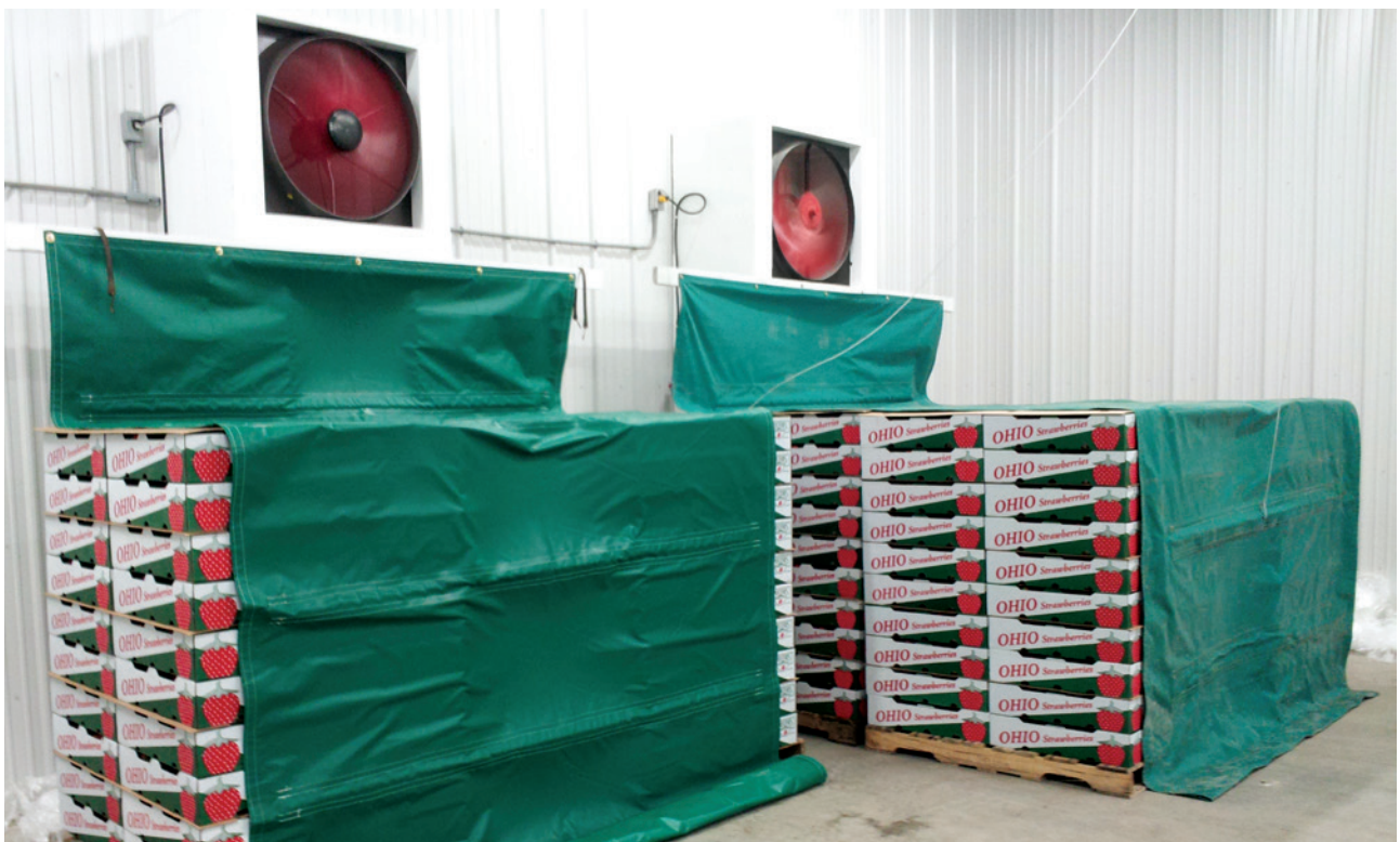
Figure 5. Simple Forced-Air Cooling System. Photo credit: Polter's Berry Farm, Ohio
