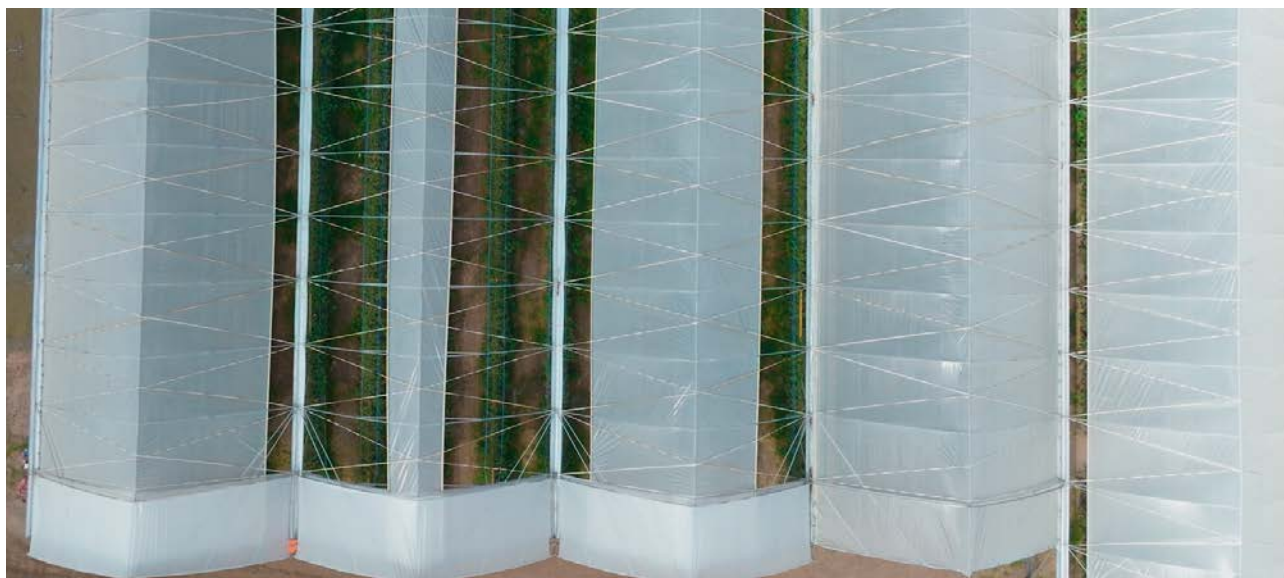
Aerial view of the Total Vent showing the polythene rolled to a range of venting positions. Photo credit: Haygrove
