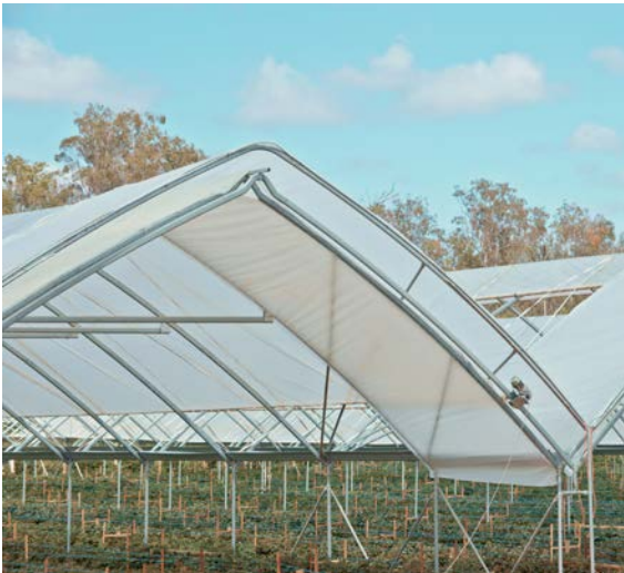
Total Vent is mechanised by electric motors, minimising the labour requirement and giving a high degree of flexibility to manage the growing environment. Photo credit: Haygrove
