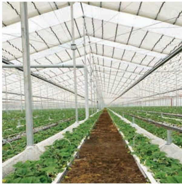
**Figure 3. On a hot day the roof is opened 50cm in each bay to allow venting, while blocking UV**
