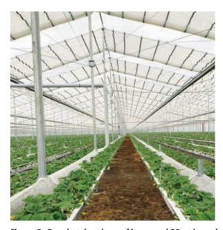
Figure 3. On a hot day the roof is opened 50cm in each bay to allow venting, while blocking UV
