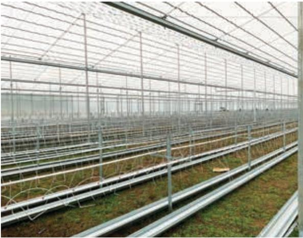
**Figure 2. Table tops under construction, showing the diffuse roof material**
