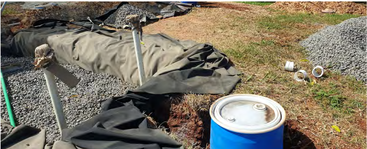
Artificial wetland reedbed under construction at Wollongbar. Photo credit: Diana Unsworth
